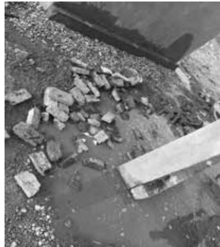
Figure 5 testing walls submerged with water
