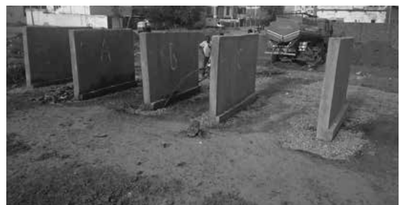
Figure 6: The constructed walls
