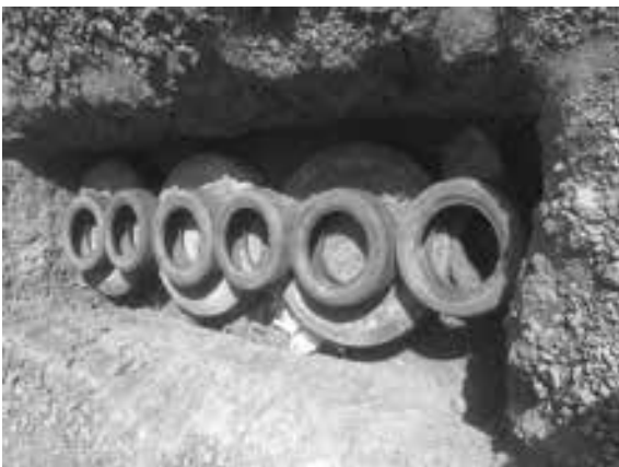
Figure 3 : Tyres filled with soil.
